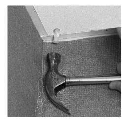
Once the anchor is installed, fully screw the eye-screw in untill the threads are no longer visible. Doing so will ensure the butterfly anchor opens on the other side.
